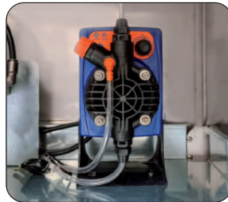
Detergent dosing pump (standard)
